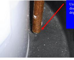
Unit C: The TPR valve discharge pipe drains to the drip pan...
