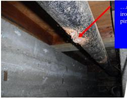
...as well, the older cast iron waste piping shows pin-hole leaks...
