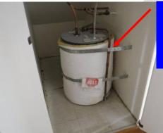
...and the seismic straps may not be over insulation blankets...
