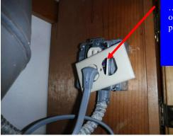
...the kitchen exhaust fan outlet has a loose cover plate...
