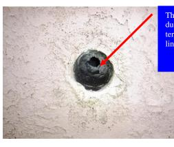
The D Unit clothes dryer duct lacks an exterior terminal and is packed with
