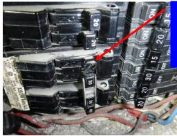
Unit C: A breaker toggle handle is damaged, the panel has two different models of breaker...
