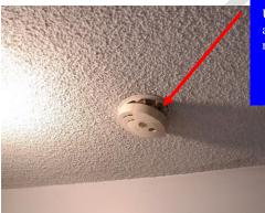
Unit C: The hall smoke alarm battery has been removed...
